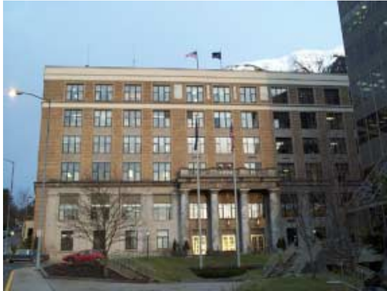
The Alaska State Capitol Building in Juneau
